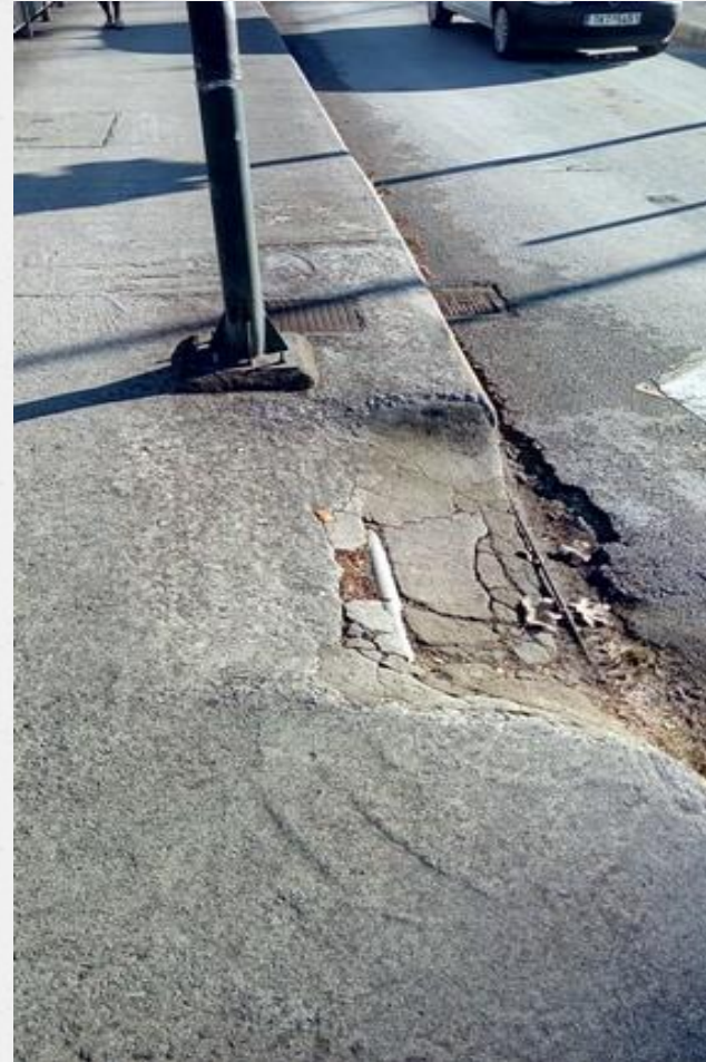
Damaged ramps
